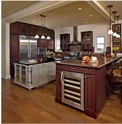
Wired up: Structured wiring makes your home one giant, functioning device. So your refrigerator, stove, microwave – and wine fridge – all are on the same page. NAHB
